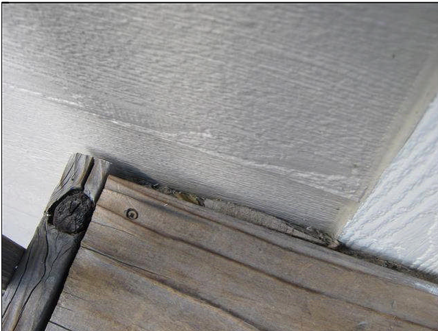
2.4 Item 5(Picture) Missing Flashing
