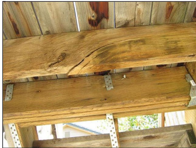
2.4 Item 4(Picture) Cracked Joist
