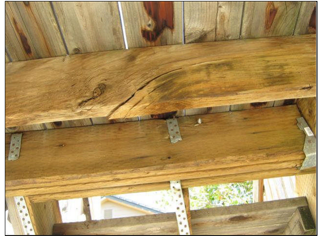
2.4 Item 4(Picture) Cracked Joist
